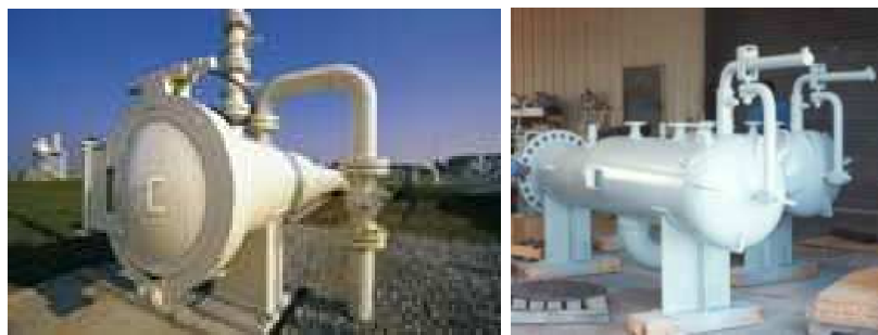
Figure 9: Pig Launcher, Receiver
