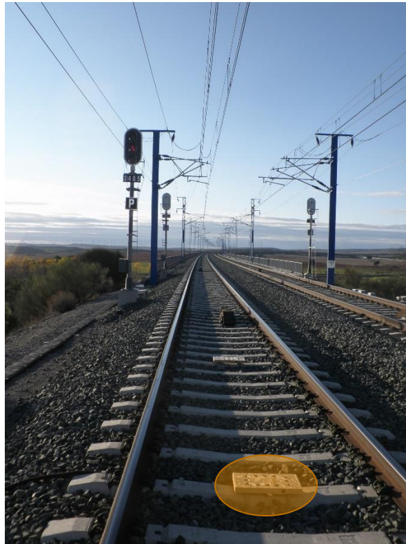
Figure 41 Bombardier ERTMS Level 2 High Speed Eurobalise © Bombardier, from press release 272
