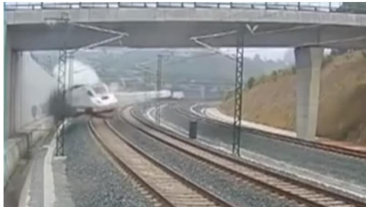
Figure 40 Santiago de Compostela derailment in Spain July 24 th 2013. 79 dead, 140 injured The conclusion from this derailment in Spain was to incorporate automatic braking systems that would avoid derailment accidents based on speed even with driver error by “installation of three balises on 1.9 km of the approach to Santiago to enforce speed limits of 160, 60 and 30 km/h” 270 .
