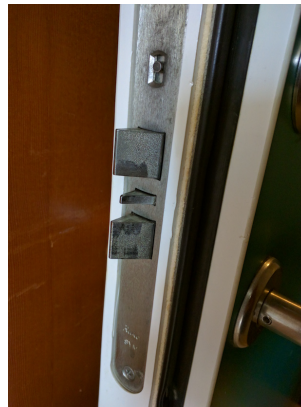
Figure 3.8: Latch bolt lock type.
