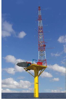
Figure 2.2: FINO 1 mast with wind sensors from 33 m to 100 m
