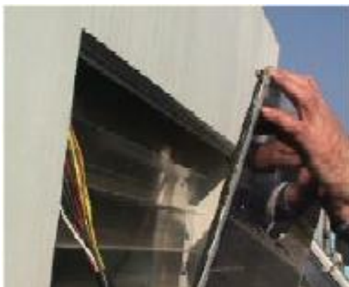
Figure 10.1: Left: A photo of the fins inside the air gap in the BIPV module[Christ 2001]. Right: A scheme showing the forced air flow in the gap.
